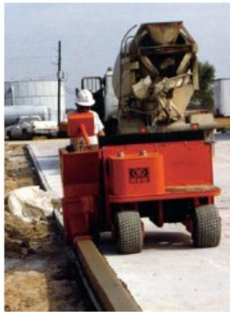
Between centers pour, kerb & gutter, valley ribbon, etc.
